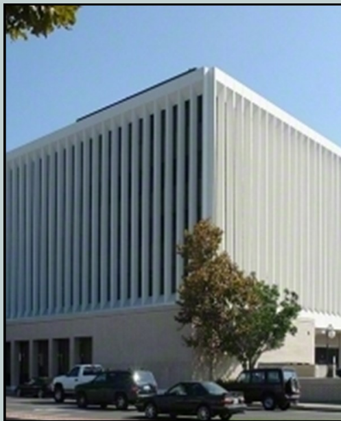
Southern California Edison incentive pays 19% of project cost to install VFD Rotary Screws solution
